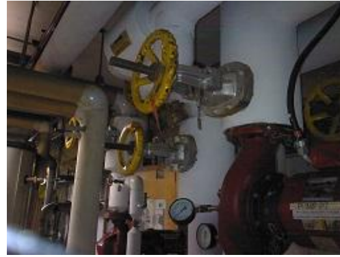
Figure 14 Conventional image of the same bare valve bonnets.
