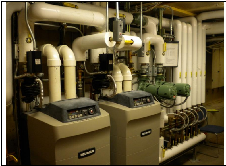
Figure 3. Diane Building (22) Boiler Installation
