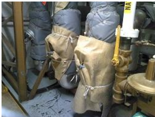
Figure 14 This is a conventional image of the same strainers covered by cloth.
