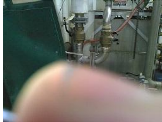
Figure 22 Conventional image of the same piping and valves.
