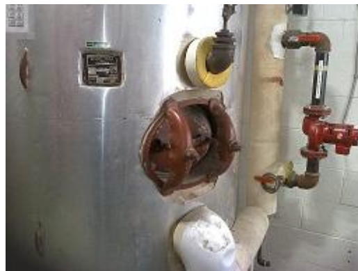
Figure 30 Conventional image of the same access hatch and piping.
