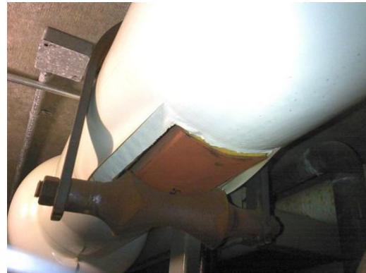
Figure 70 Conventional image of the same roller support.
