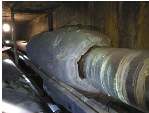
Figure 84 Conventional image of the same exchanger.
