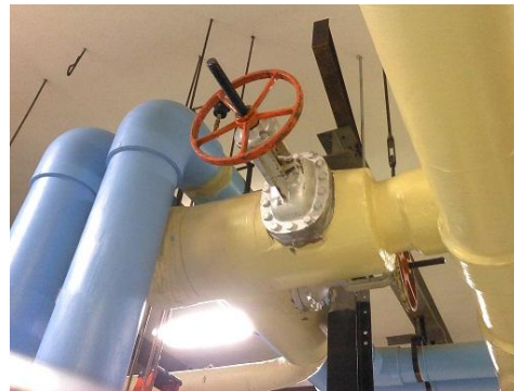
Figure 4 This is a conventional photo of the same exposed valve bonnet.
