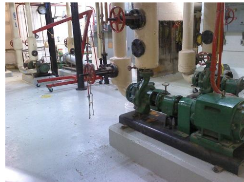
Figure 28 Conventional image of the same pump.
