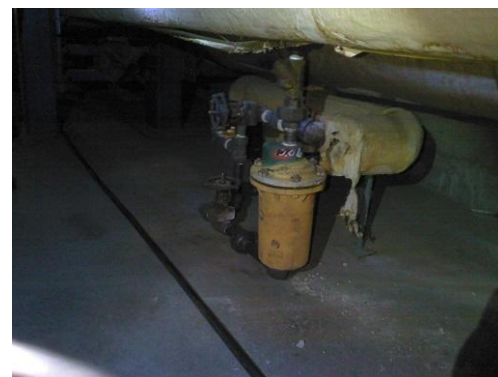
Figure 64 Conventional image of the same steam trap.
