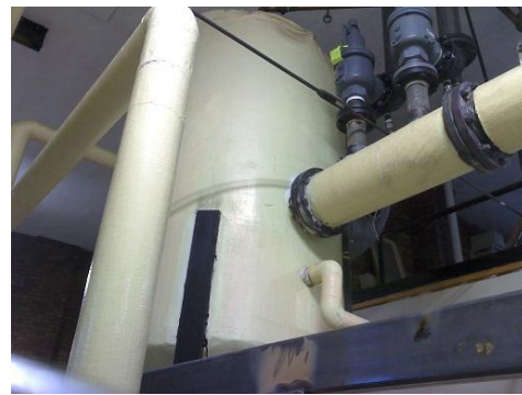
Figure 10 This is the conventional image of the same bare flange and piping.
