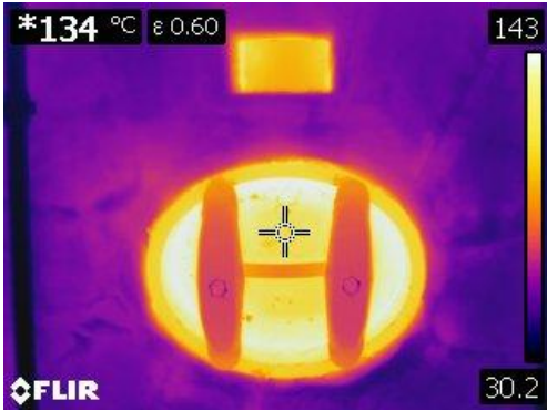
Figure 13 Thermographic image of a bare manway at 134° C or 134 °F
