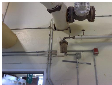
Figure 12 This is the conventional image of the same steam trap.
