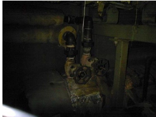
Figure 74 Conventional image of the same valves.
