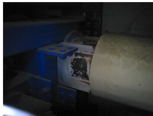
Figure 60 Conventional image of the same pipe rack support.
