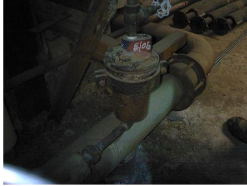
Figure 94 Conventional image of the same steam trap.
