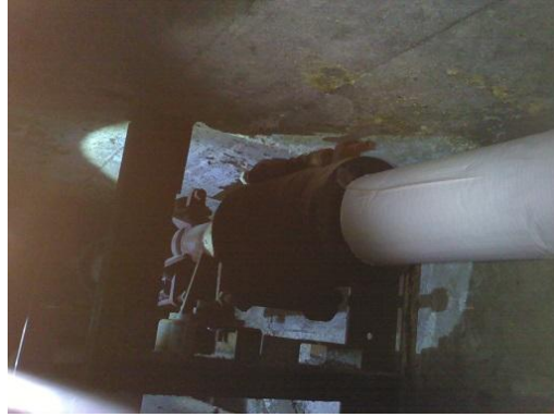
Figure 106 Conventional image of the same expansion joint.
