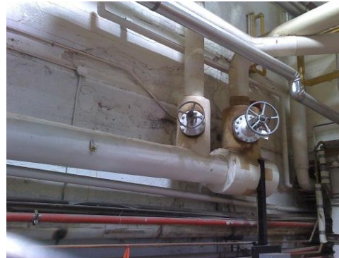
Figure 48 Conventional image of bare valve bonnets. Note the canvas is burnt due to exposure to high temperatures.
