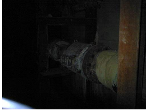
Figure 112 Conventional image of the same expansion joint.
