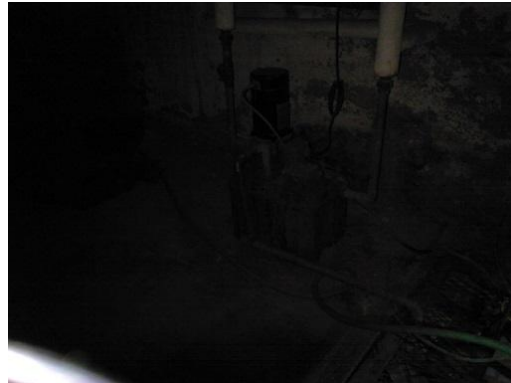
Figure 90 Conventional image of the same sump pump.
