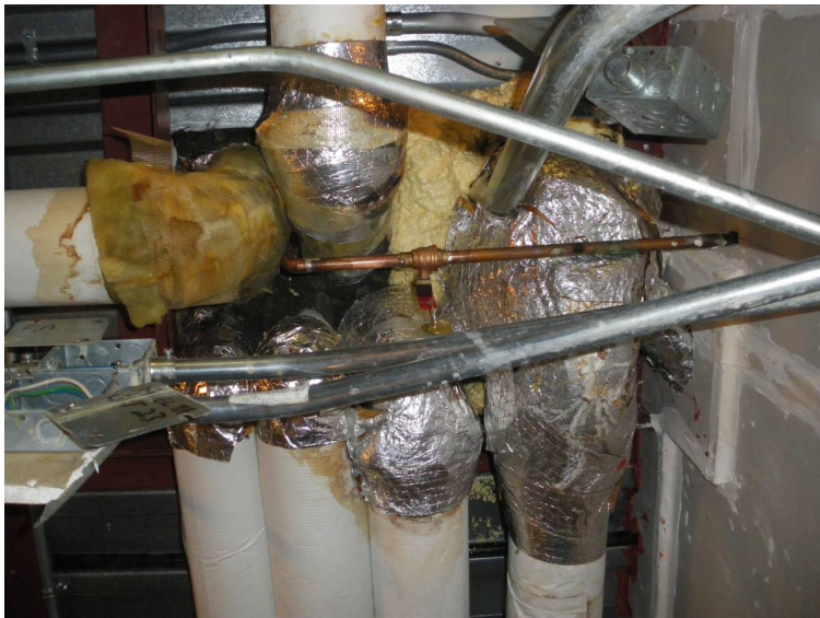
Sweating pipes in a medical building in Vancouver. Note insufficient space adds to the problem.
