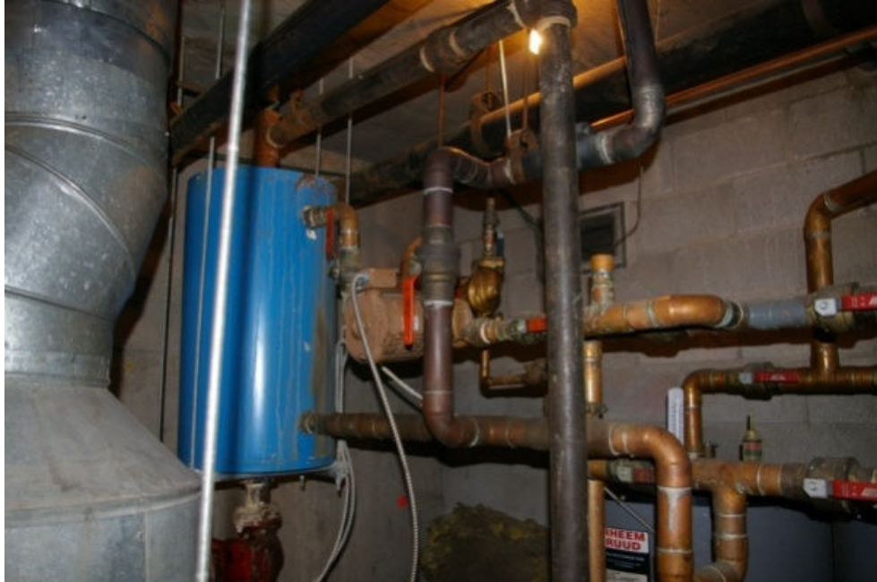
Photo 2 Detail showing un-insulated hydronic distribution system and heat exchanger for domestic hot water system
