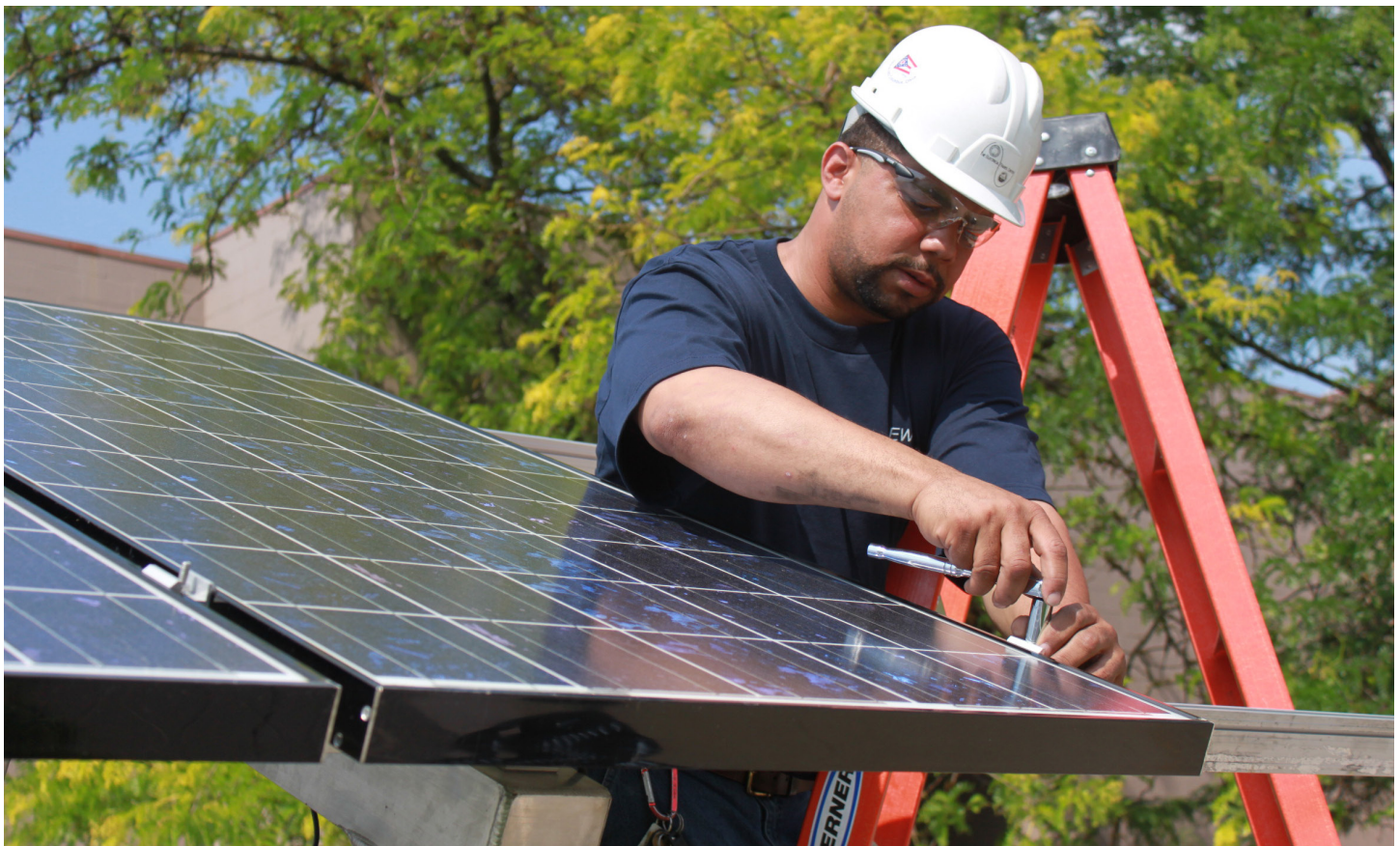
IBEW Local 683 worker installing solar panels.
