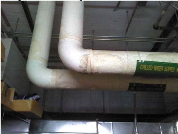
Chilled Water Piping with Moisture
