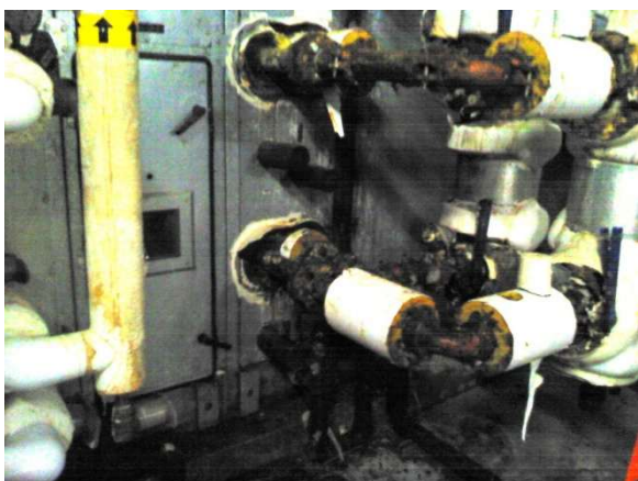
Missing Insulation, significant energy loss – condensation issue & Corrosion Under Insulation (CUI)
