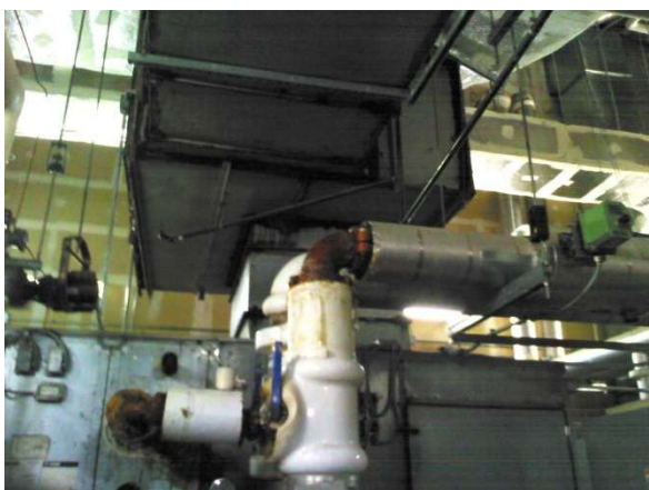
Missing Thermal Insulation, significant energy loss - condensation issue & Corrosion Under Insulation (CUI)
