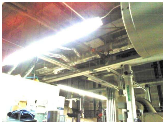
Issues with Ductwork Insulation Energy Loss - condensation issue & Corrosion Under Insulation (CUI)
