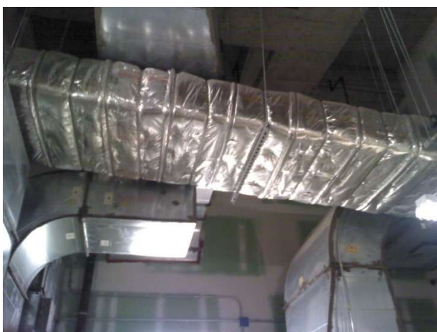
Kitchen Exhaust Fire Protection Insulation –
