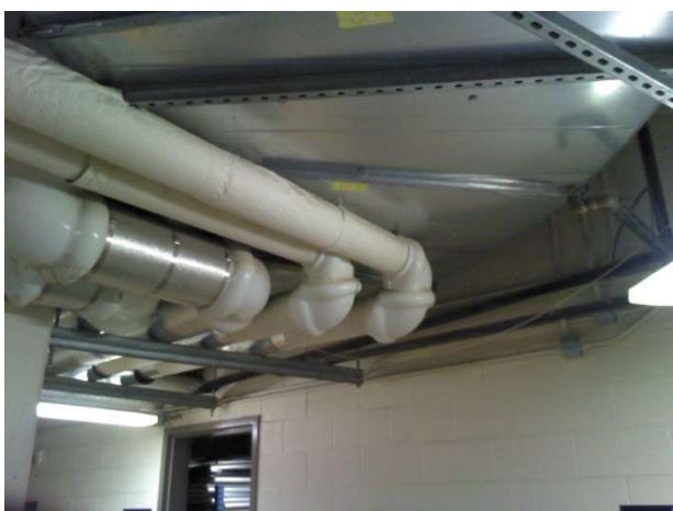
Improper Thermal Insulation Installation, allowing significant energy loss, due to installation issues
