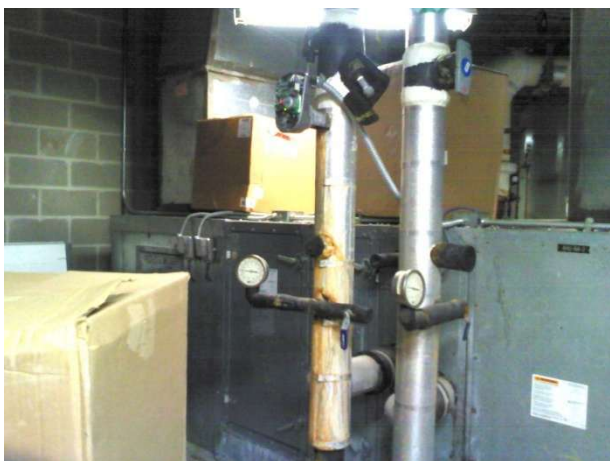
Inadequate Chilled Water Insulation in Insulation allowing moisture condensation
