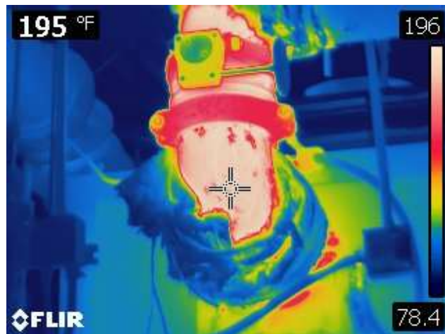
Infrared Image of Uninsulated Hot Water Heating Piping with significant energy loss
