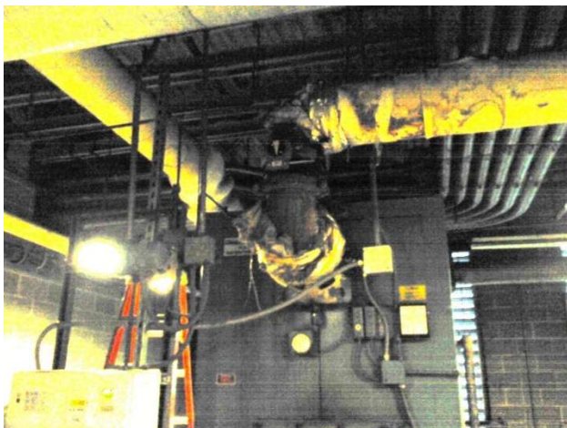
Uninsulated Hot Water Heating Piping with Heating Piping with significant energy loss
