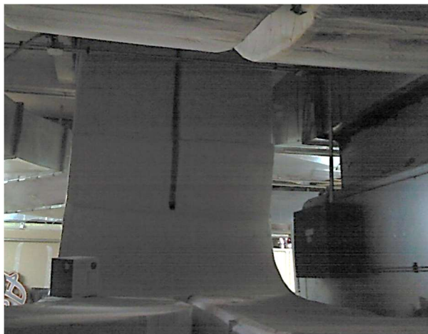
Insulated Ductwork in Mechanical Room
