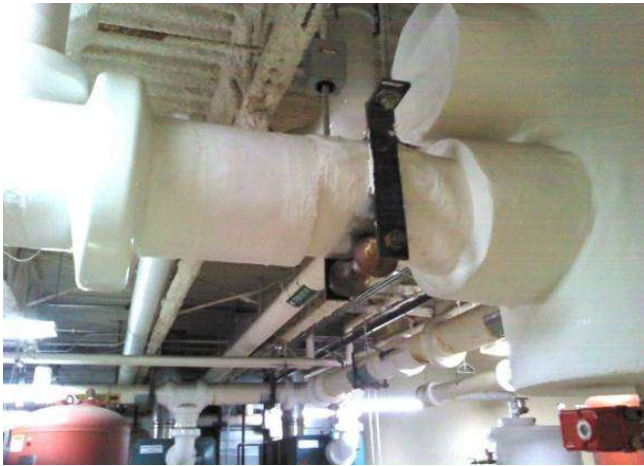
Improper Support with Compromised Insulation
