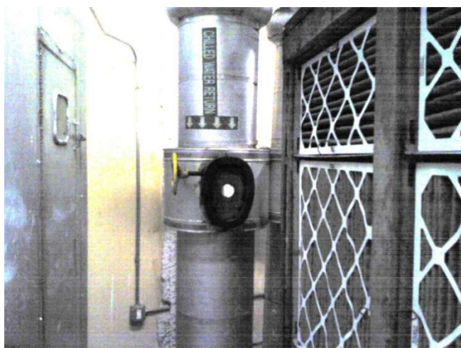
Inadequate Chilled Water Insulation
