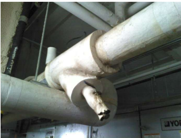
Chilled Water Piping in Mechanical Room
