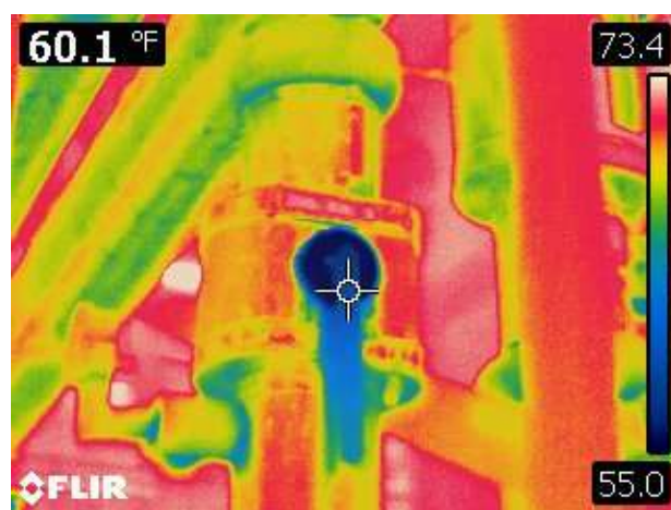
Infrared Image of Inadequate Chilled Water allowing condensation leading to mold growth
