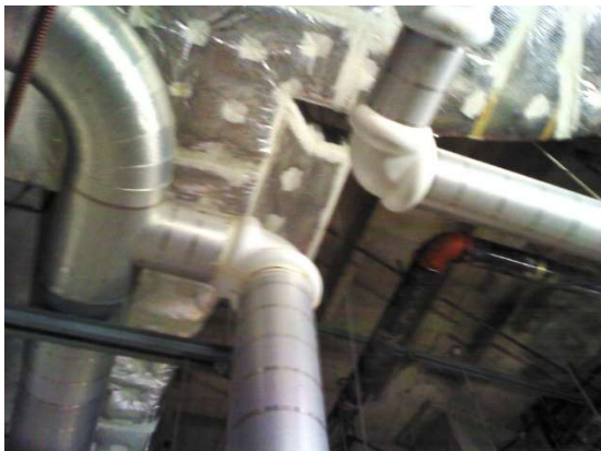
Issues with Ductwork Insulation – Energy Loss
