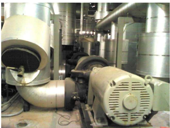
Thermal Insulation Issue, allowing energy loss – condensation issue & Corrosion Under Insulation (CUI)
