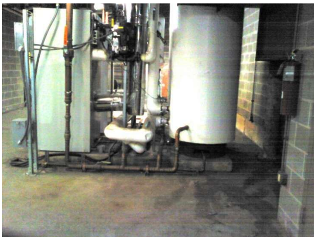
Missing Domestic Hot Water Insulation
