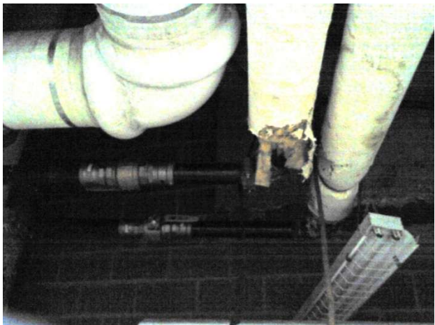
Compromised Insulation due to Improper Support & Missing Insulation
