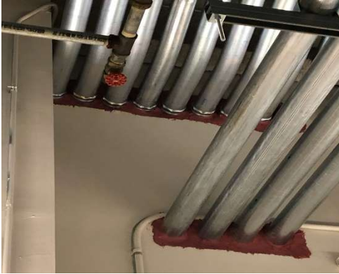
Firestopped Conduit in Wall
