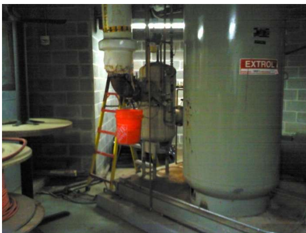
Uninsulated Hot Water Heating Piping Heating Piping with significant energy loss
