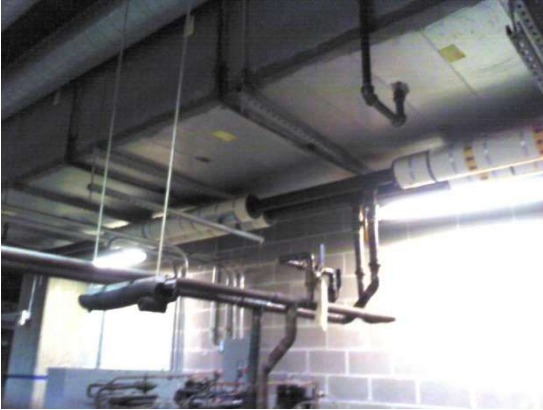
Missing Insulation on Food Service Recovery Piping System
