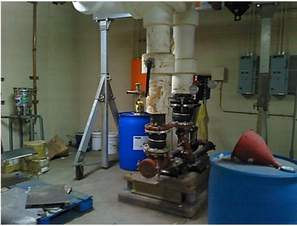
Missing Insulation with Significant Heat Loss
