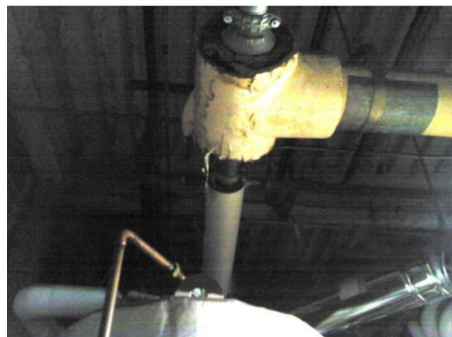
Missing Domestic Hot Water Insulation Contributing to fluid temperature drop
