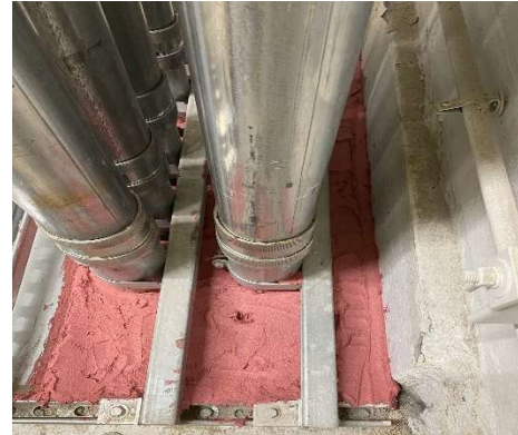
Firestopped Conduit in Floor
