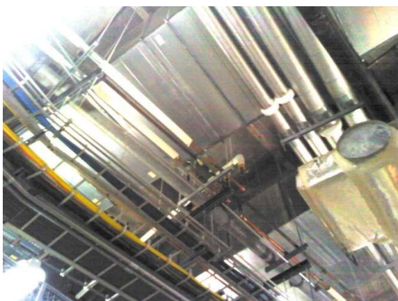
Missing Thermal Insulation, allowing significant energy loss
