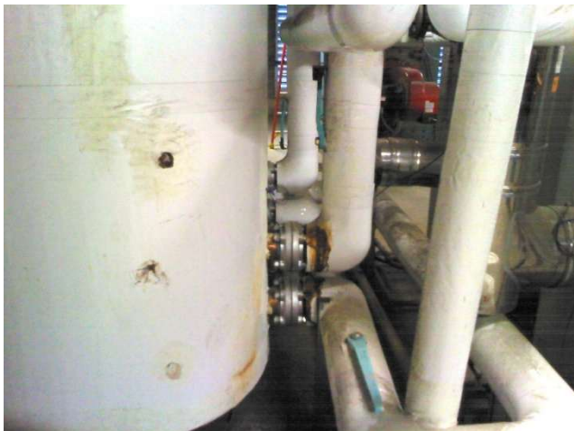
Missing Domestic Hot Water Insulation
