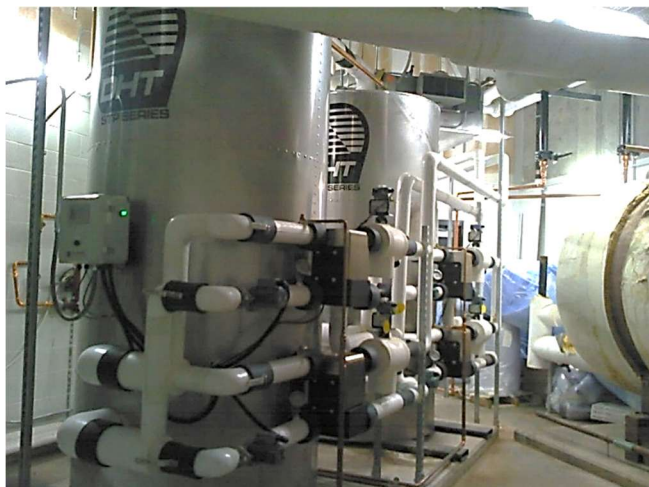
Domestic Hot Water Tanks & Piping
