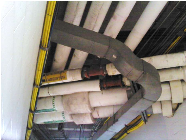
Missing Heating Hot Water Insulation
