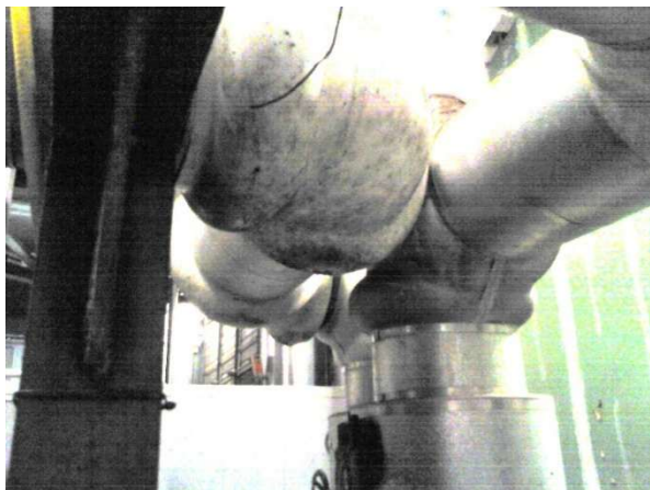
Chilled Water Piping without proper vapor barriers, allowing moisture accumulation
