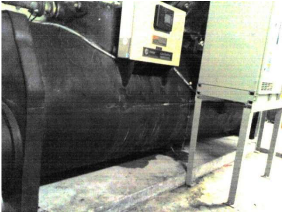
Compromised Elastomeric Foam Insulation
